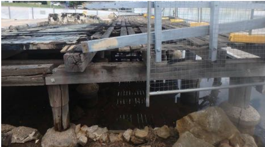
Figure 19: View of piles, beams, square headstocks, transverse planks (just visible to LHS) and deck planking, facing W. (Cosmos Archaeology Pty Ltd, 29 th November 2017)
