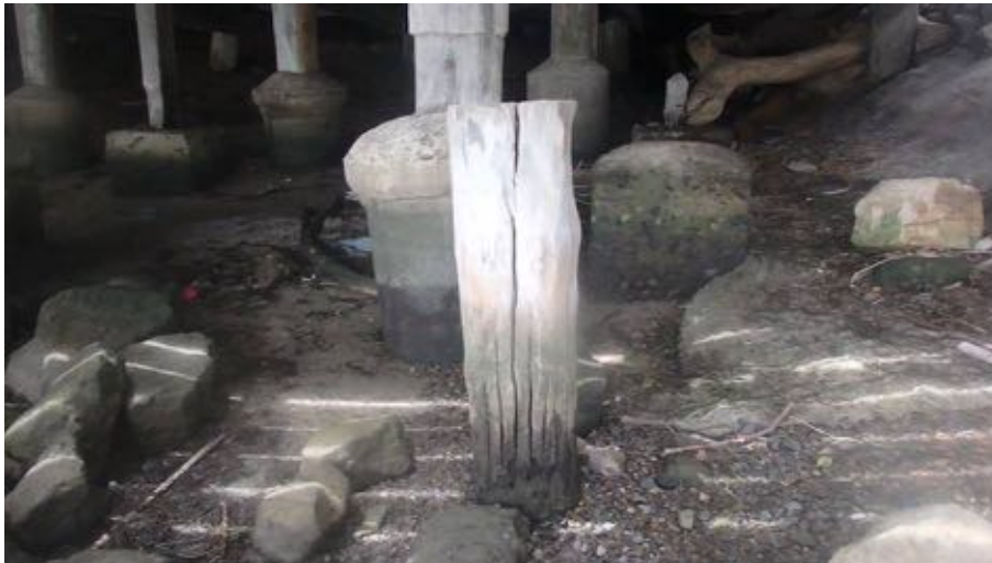
Figure 25: Standing pile stump of relatively good condition towards western side of the wharf, facing S. (Video Nowra Wharf 014, still image taken at 00:13).
