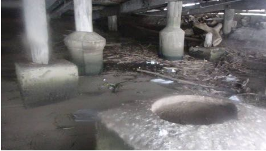
Figure 20: Three square concrete footings, two with cut piles and one without, in contrast to the round concrete jackets, facing SW. (Video Nowra Wharf 007, still image taken at 01:12)
