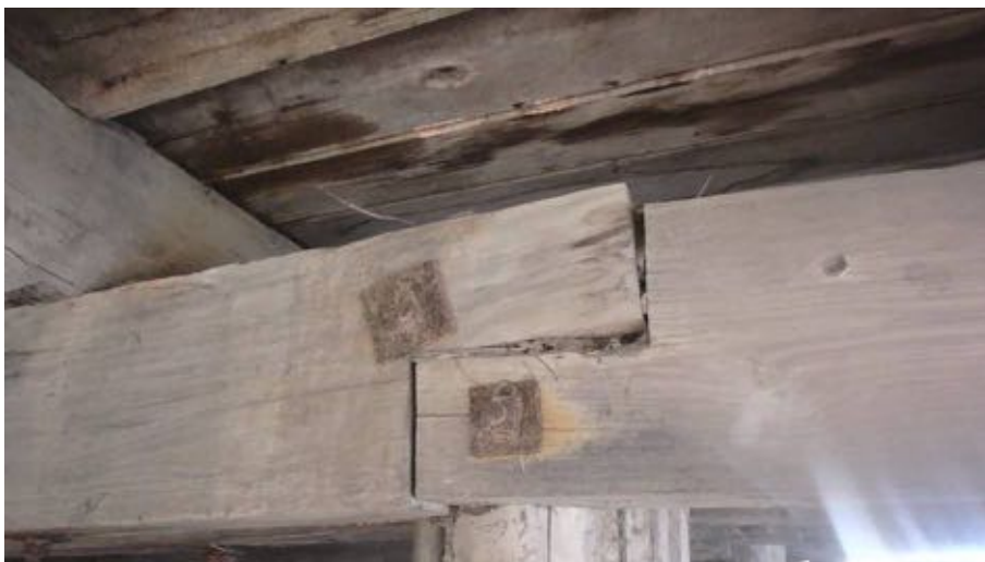
Figure 15: Rectangular beam with half-lap scarf joint with bolts, facing WSW. (Video Nowra Wharf 002, still image taken at 01:11)
