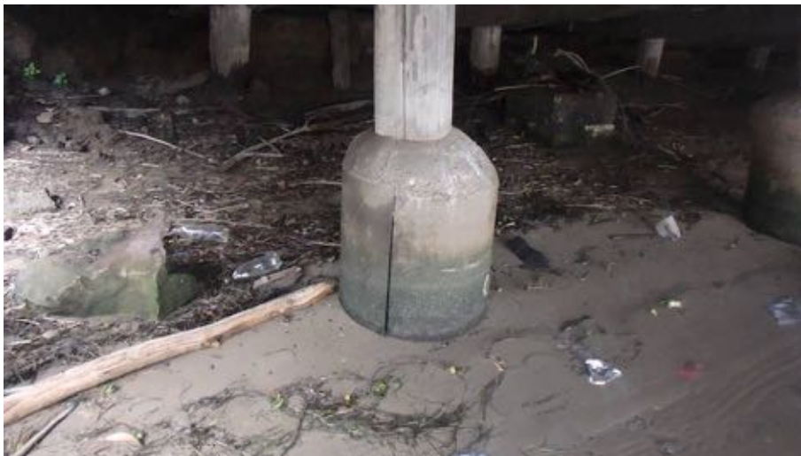
Figure 13: Round concrete jackets without shaping at the top, possibly indicating that they are newer additions, facing SSW. (Video Nowra Wharf 001, still image taken at 01:33)
