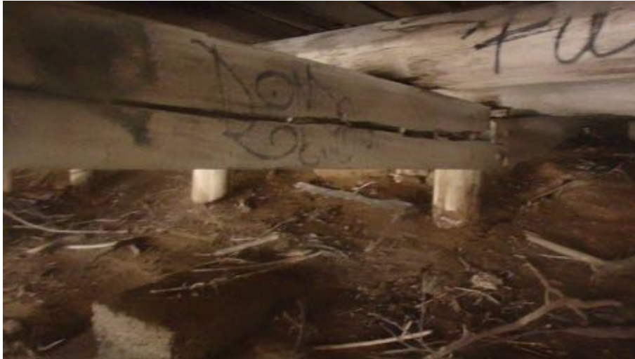
Figure 16: Split along the centre of a beam. (Video Nowra Wharf 10, still image taken at 00:53)
