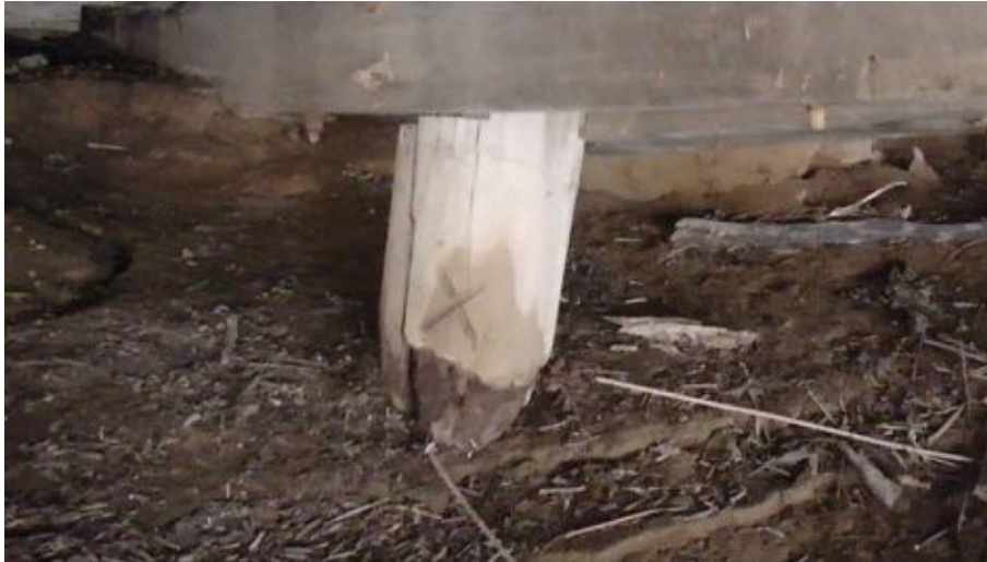
Figure 14: One of the piles showing evidence of a split, facing SSW. (Video Nowra Wharf 005, still image taken at 01:49)
