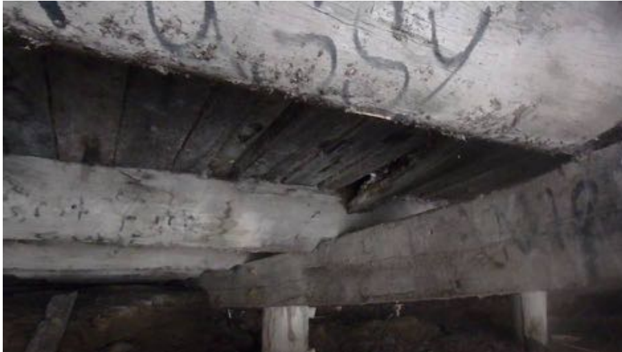
Figure 18: View of the round piles, rectangular beams, round headstocks and transverse planks, facing SSW. (Video Nowra Wharf 004, still image taken at 01:06)
