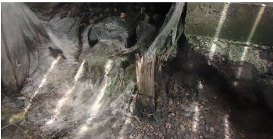
Figure 28: Degraded pile stump, being the smaller identified on the western side of the wharf, facing WSW. The larger of the two piles is visible on the RHS of the image. (Video Nowra Wharf 014, still image taken at 00:25)
