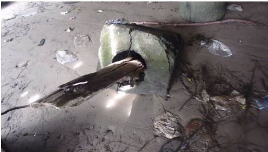
Figure 21: Toppled square concrete footing with degraded pile remains and round footing in background, facing SSE. (Video Nowra Wharf 005, still image taken at 01:21).
