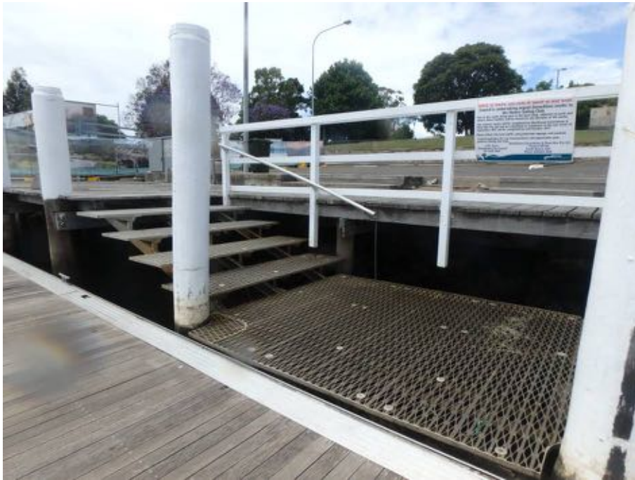
Figure 35: Wide steel grill stairs from the wharf to floating pontoons, facing SE. (Cosmos Archaeology Pty Ltd, 29 th November 2017)
