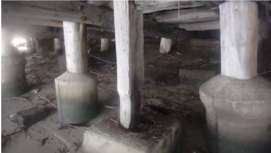
Figure 22: Standing pile in square footing that has snapped along its length, facing SSE. (Video Nowra Wharf 010, still image taken at 00:26)
