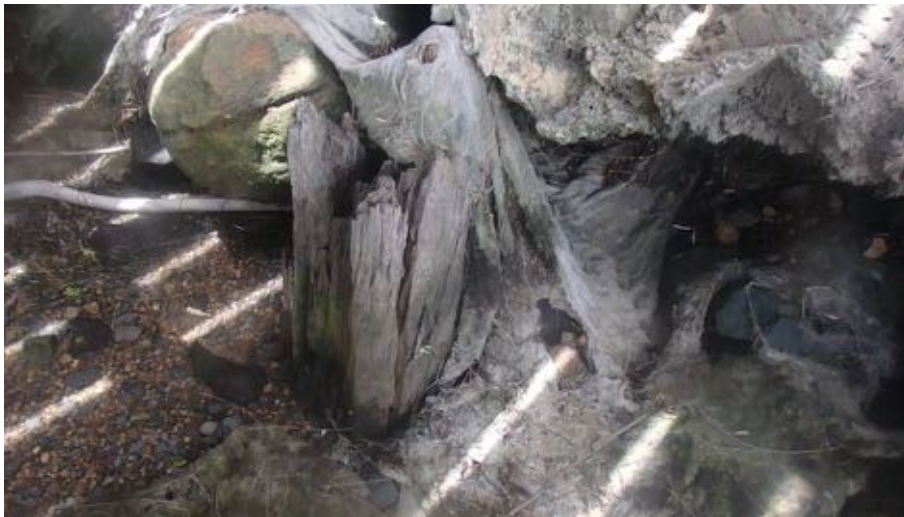
Figure 27: Degraded pile stump, being the larger identified on the western side of the wharf, facing SW. (Video Nowra Wharf 014, still image taken at 00:30)
