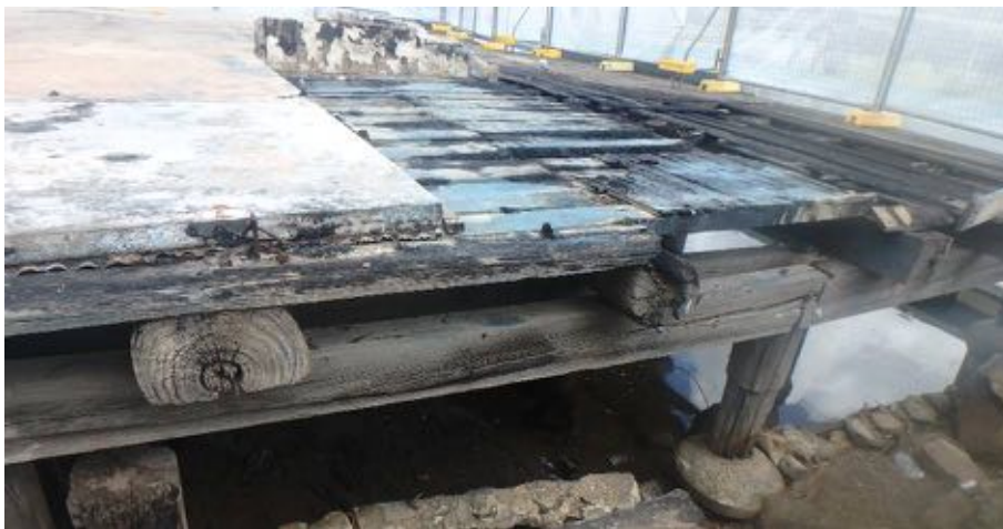
Figure 17: View of the ends of three timber headstocks – from left to right there is one crescent-shaped, one round and one square headstock, facing WNW. (Cosmos Archaeology Pty Ltd, 29 th November 2017)
