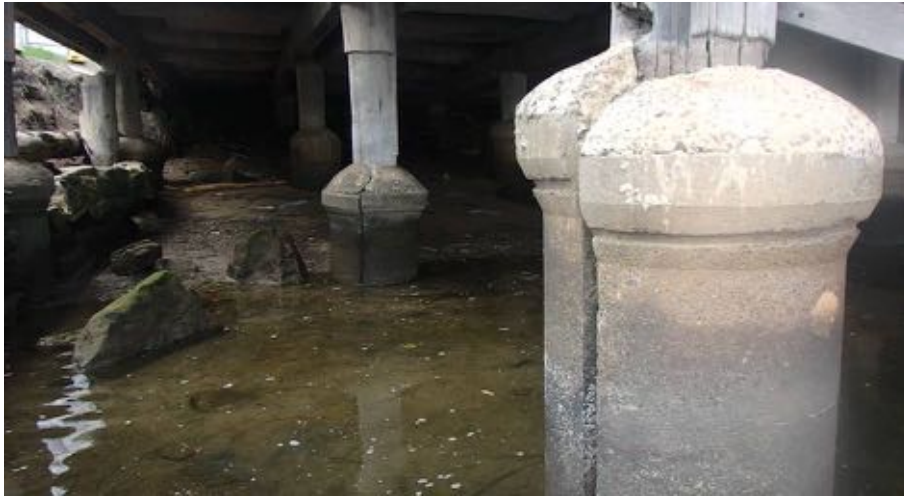
Figure 12: Round concrete pile jackets, showing the split and sliding which likely indicates damage, facing SSW. (Video Nowra Wharf 001, still image taken at 00:14)
